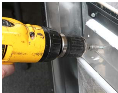
Figure 4: The screws securing the bracket and the insulating material should be driven in at slight downward angle.
