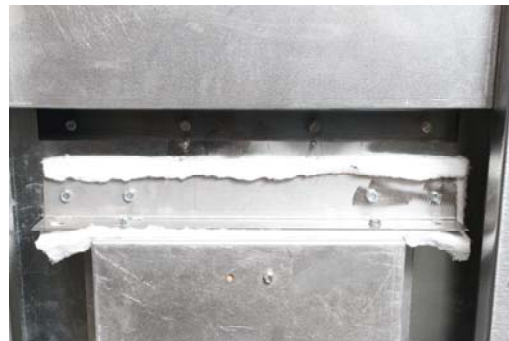
Figure 5: The insulation/bracket assembly is shown in place at the rear of the burner chamber.
